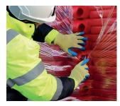
The plastic wrap is easily removed by carefully running a knife through the shrink wrap material.
