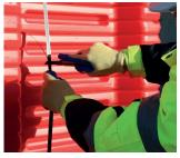
The plastic banding straps can be cut carefully with a knife.
